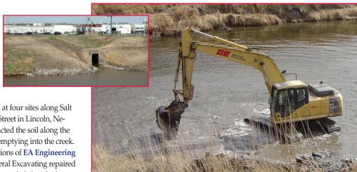
maintenance work to be performed at four sites along Salt Creek from 20th Street to Superior Street in Lincoln, Nebraska. Erosion and time had impacted the soil along the banks and the drainage structures emptying into the creek. Following the design and specifications of **EA Engineering Science and Technology, Inc.**, General Excavating repaired miscellaneous concrete structures, regraded sloughed banks, placed rip rap and associated work.
