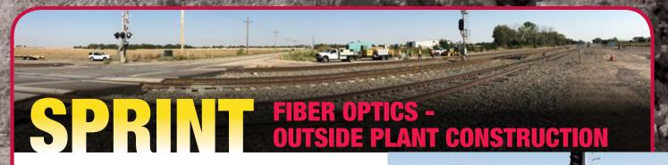
INSTALLATION OF FIBER OPTICS in a railroad right-of-way provide a unique set of challenges as trains can cruise by at speeds approaching 70 miles per hour. Such is the case on a recent General Excavating's job site installing innerduct and fiber optics for *SPRINT* in a Union Pacific right-of-way near Grand Island, Nebraska. Before crew members are allowed on site, they must become *UNION PACIFIC* Fiber Optics Safety Trained. This training is an essential part in understanding the
